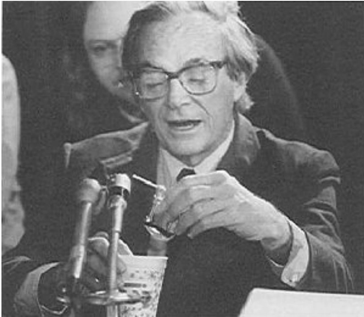
Feynman O-ring Ice-Dunk Experiment
